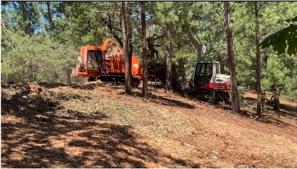
Excavator feeding cut brush and small trees into high-horsepower chipper
