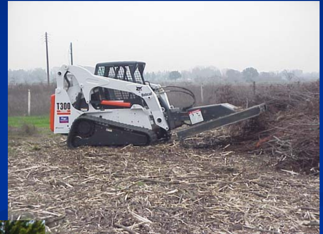
Using Bobcat to break down biomass (2004)
